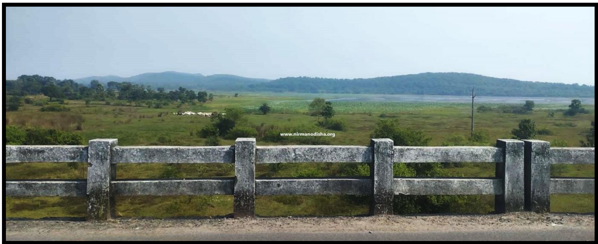
A part of the Khandak nala joining the Anshupa lake, as seen from the bridge. Mahanadi flood water occasionally enters the lake also through this route.
