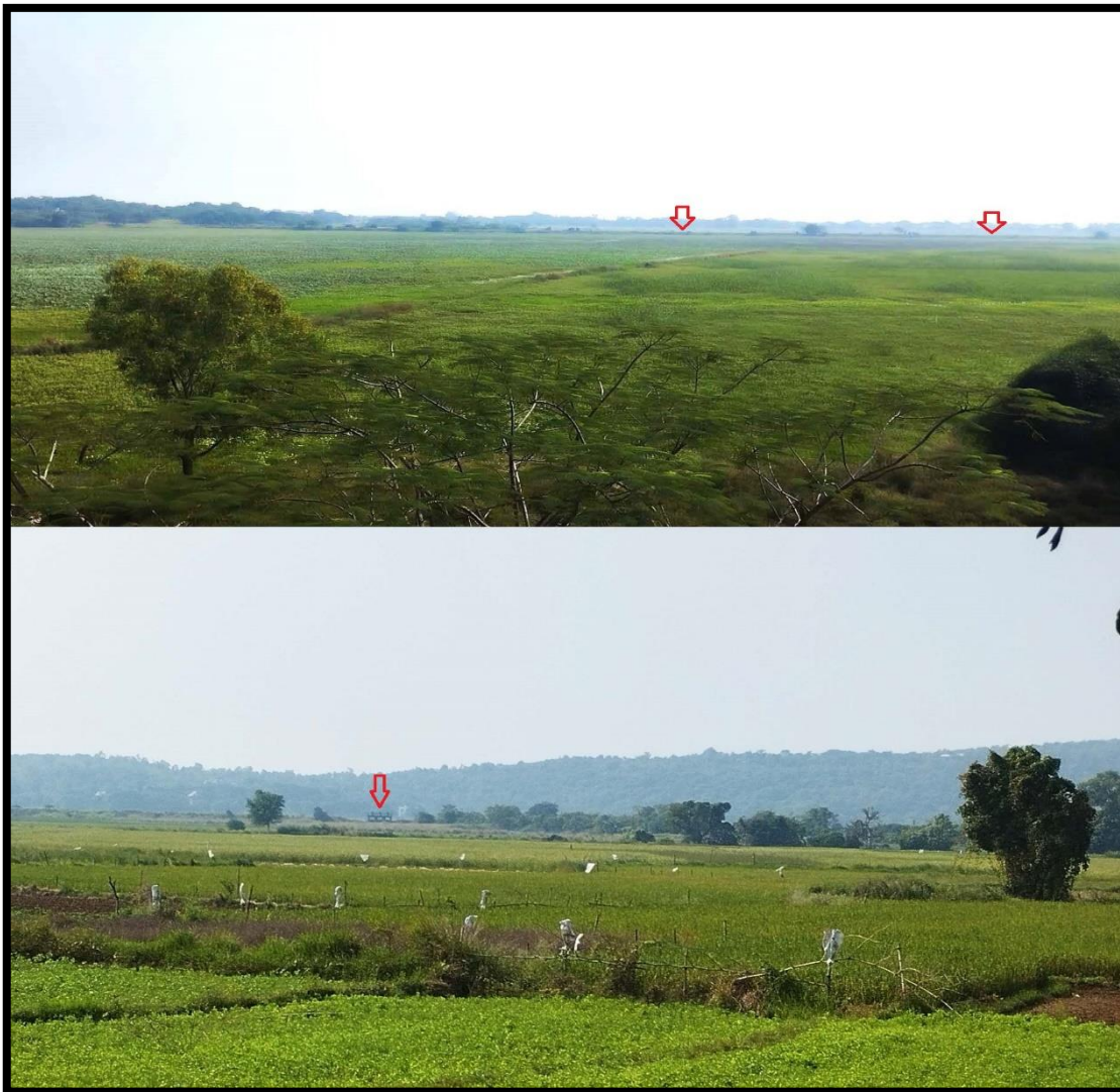
The Dahaliani embankment from the lake side (upper) and Subarnapur side(lower) as marked by the red arrows. The arrow on the lower image shows the sluice gate.
