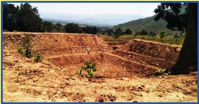
(Left) The CFRR title for Poduchuan signed by government authorities. (Right-upper) Farmers like Tamana Pidisika could grow sunflower & other crops in their fields with confidence & care after their land rights got recognized and they were no more treated as encroachers in their own lands; (Right-lower) Percolation tanks are a part of the rain water harvesting structure being developed in Poduchuan.
